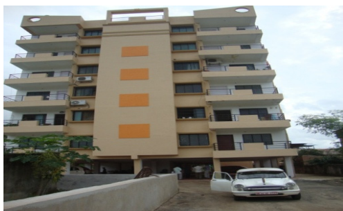
One S+6 building constructed at Ghatikia against the approved plan of S + 4 building
